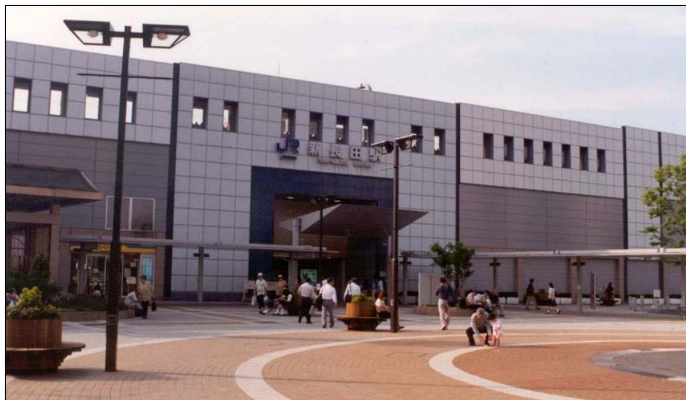
Figure 7-4: New front plaza at Shin-Nagata JR Station, June 2000
