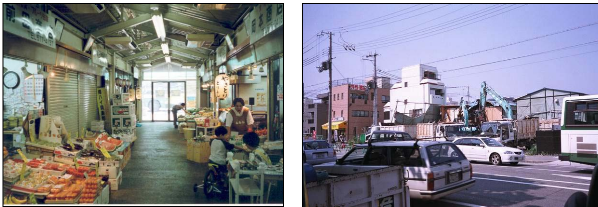
Figure 8-22: (a) Interior view of temporary arcade in July 1999; (b) Arcade demolition underway in June 2000
