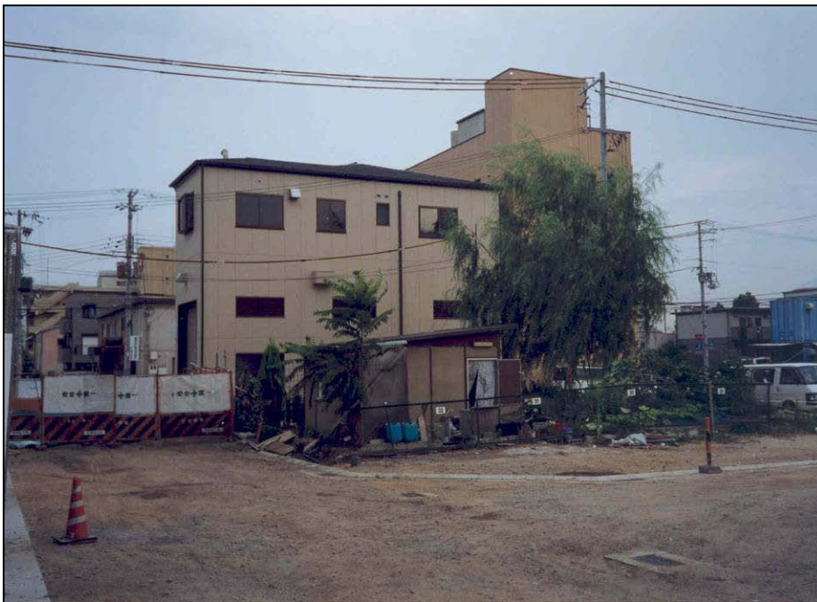
Figure 8-17: Two-story factory-house on replotted land, July 1999. Former building was partially damaged and then demolished after the earthquake. It had been located in what is a new street to the left of the new structure.
