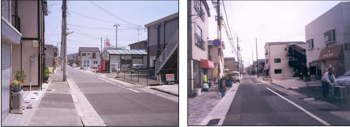
Figure 8-14: June 2000 (a) and January 2003 (b) comparisons of streetscape undergoing widening to 10 meters as part of Misuga West land readjustment.
