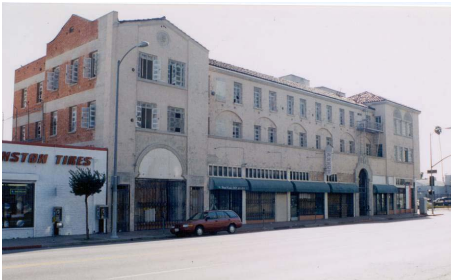
Figure 4-14: Don Carlos Building Under Reconstruction in 1999, April 1999 and March 2000
