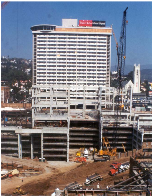
Figure 4-18: Hollywood & Highland Project Construction Underway in March 2000
