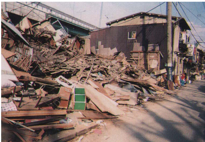
Figure 9-9: Earthquake Damage to Homes on Site of Casa Bella I and II Joint Housing
