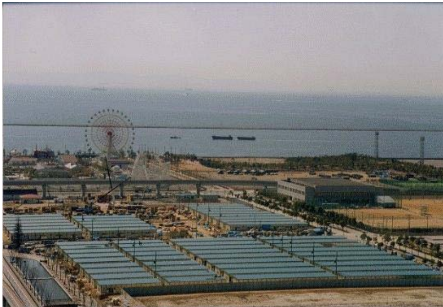
Figure 6-7: Temporary Housing Using Sea Containers, Rokko Island, March 20, 1995
