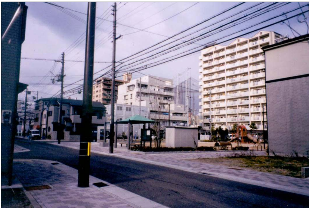
Figure 8-10: 1000 sq meter park constructed near public housing and along 10 meter widened street in Misuga West, 2003
