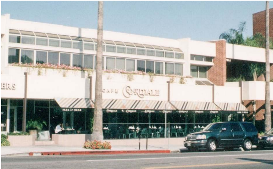
Figure 3-15: Café Cordiale, in 2-Story Portion of Scotty Building, Ventura Boulevard, 1998
