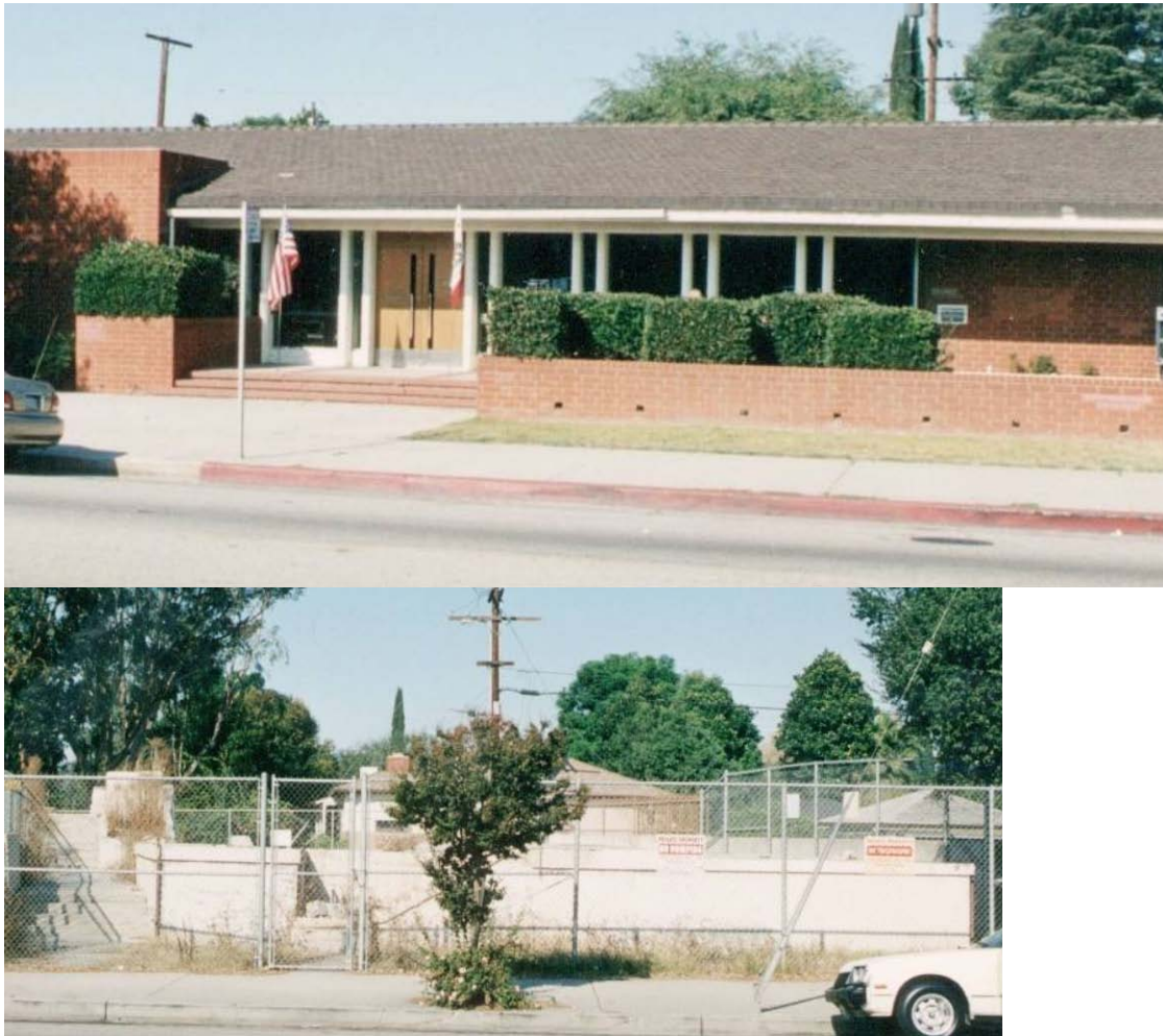
Figure 3-9: Sherman Oaks Library, and Adjacent Vacant Lot
