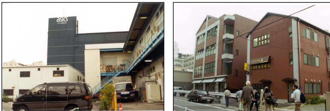
Figure 7-41: Rebuilt (a) Asics Shoe building and (b) Lion Shoe building, June 2000
