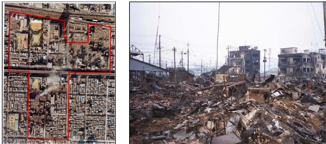
Figure 7-6: (a) Shin-Nagata South Redevelopment Area boundaries on 1995 aerial photograph (City of Kobe, 1997) and (b) Ground-level view fire-devastation in Nagata Ward (Earthquake Engineering Research Institute, 1995)
