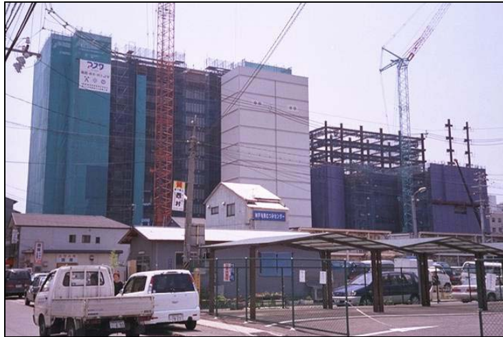
Figure 7-30: Looking south toward Wakamatsu 3 project under construction, June 2000
