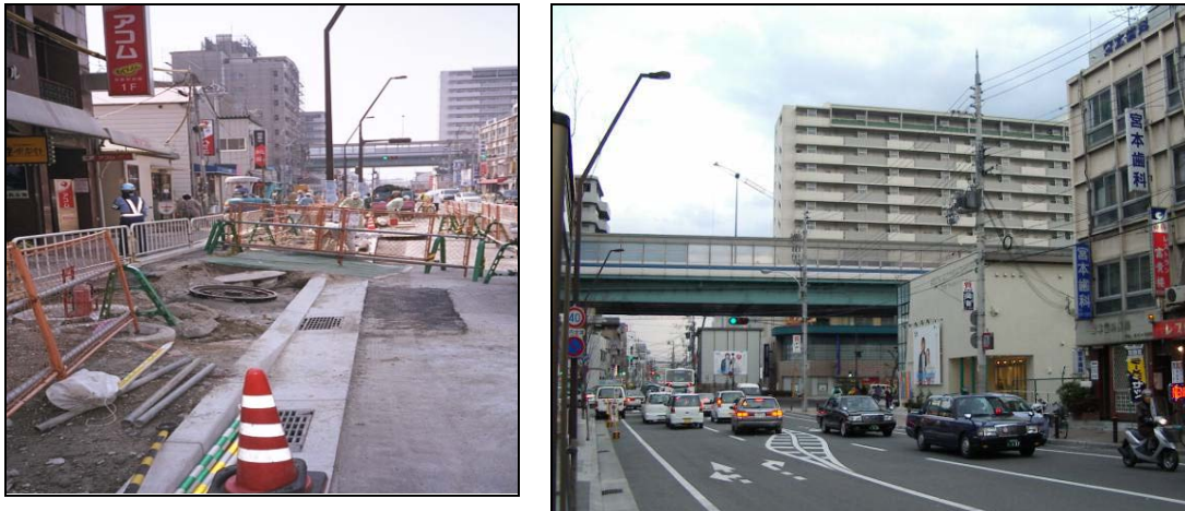
Figure 7-5: Looking south from the JR station at the subway line and Goinoike Road widening in the Shin-Nagata South area (a) underway in June 2000 and (b) completed in January 2003
