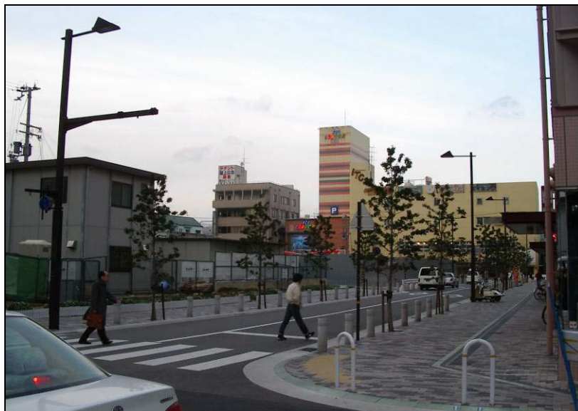
Figure 7-31: Road widening and temporary facilities in Shin-Nagata South Area No. 3, January 2003
