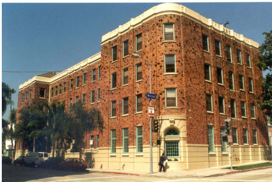
Figure 4-12: Rehabilitated Wilcox Apartments, March 2000
